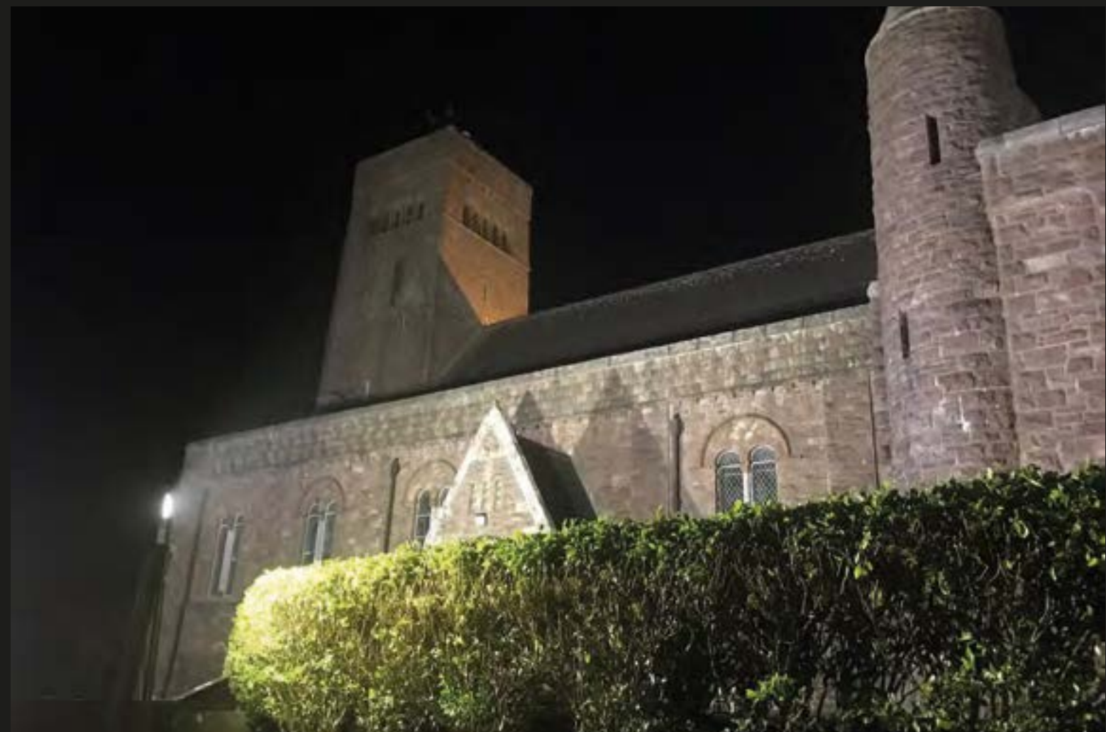
Current floodlights directed at the church with excessive white light.
