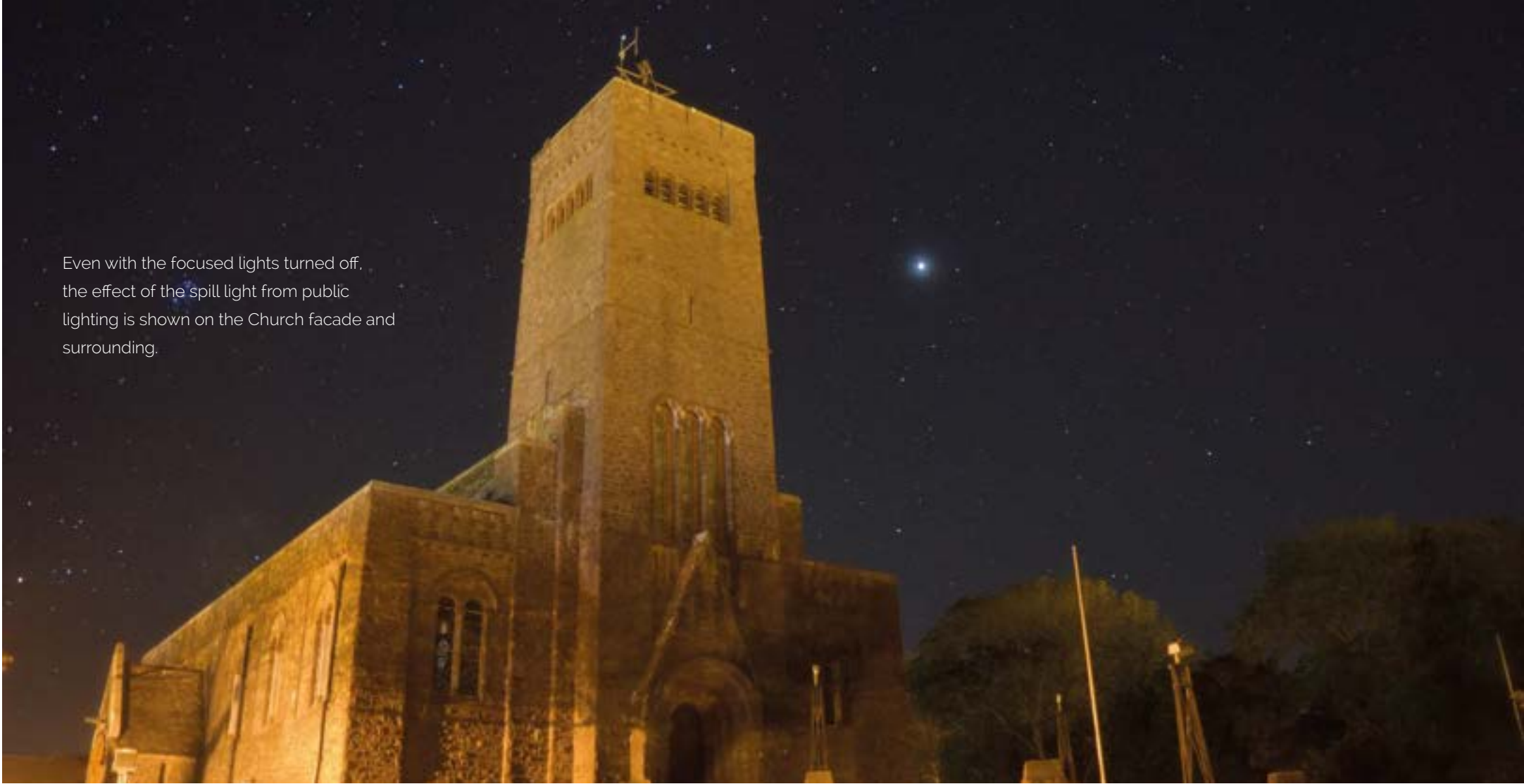
Current floodlights over illuminate the church façade causing glare to visitors and excess light at night shining into the sky
